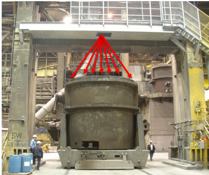
bridge over ladle transport car
